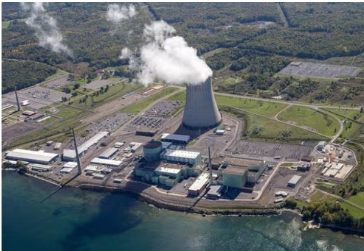
Nine Mile Point Nuclear Power Plant (source: Constellation Energy)
